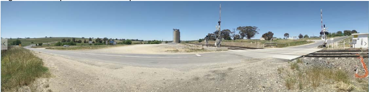
Figure 4 - View from Cunningham Road towards site showing existing ingress sited 6.5 metres from the hold line on Cunningham Road for the railway level crossing.
